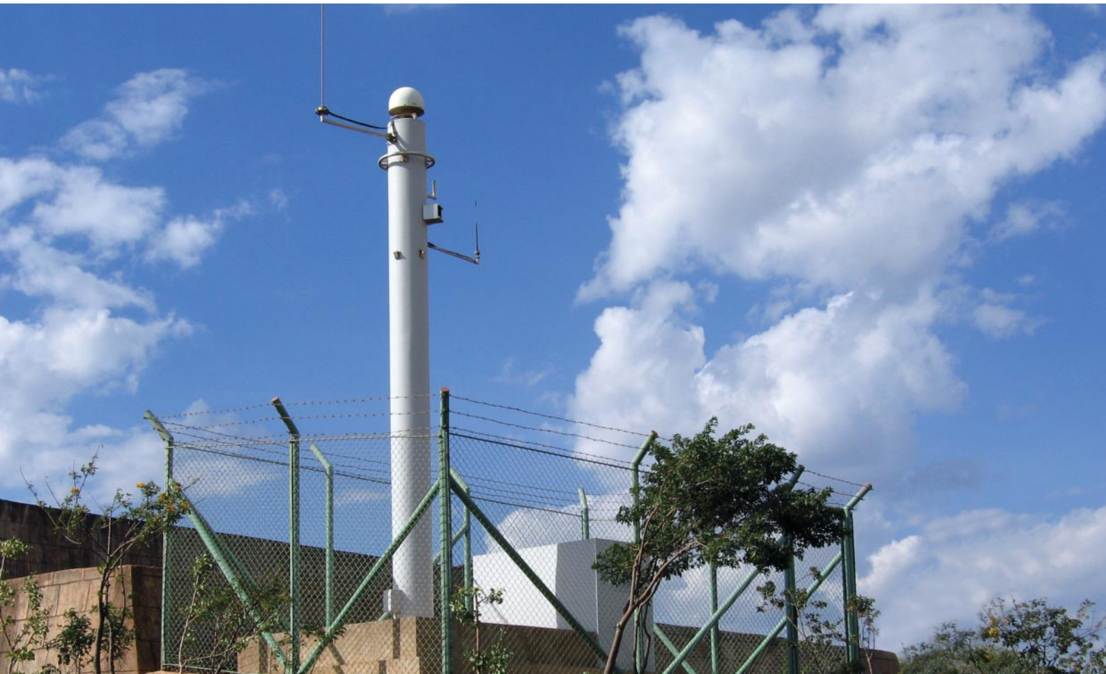
■ Horsrace branch station of Kunming GPS Reference station Network
