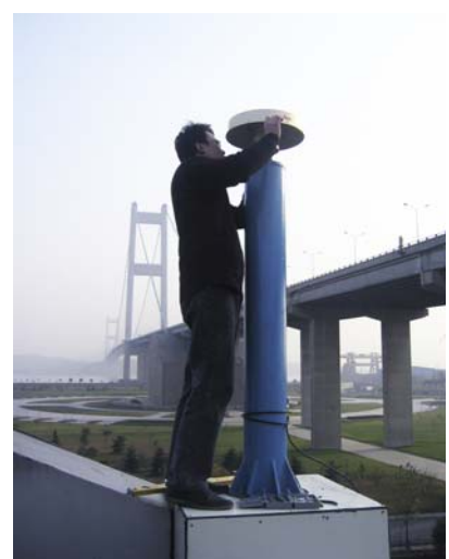
Mr. Li of Leica Geosystems partner EuroAsia installing a GPS monitoring station
