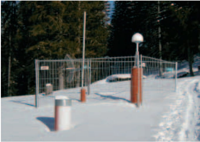
(Above): Permanent GPS station with Wireless-LAN antenna after completion
